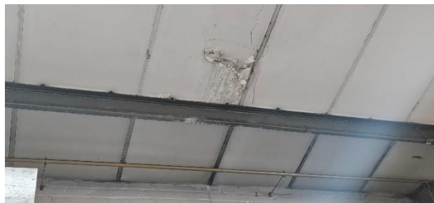
Historic water damage to asbestos roof
