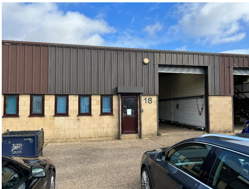
Unit 18 Staveley Way
