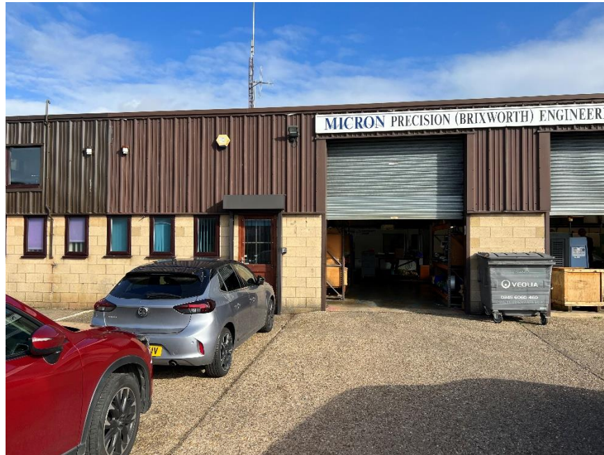
Unit 14 Staveley Way
