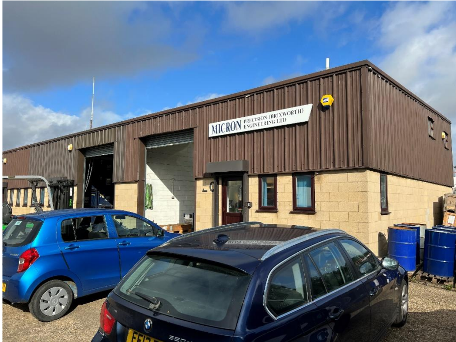
Unit 20 Staveley Way
