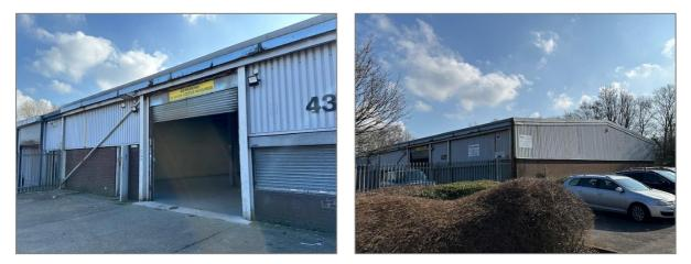
The property is of typical construction for its type and age, with steel portal frame, part brick, part steel profile clad elevations and double-skin, steel profile roof, with skylights.
